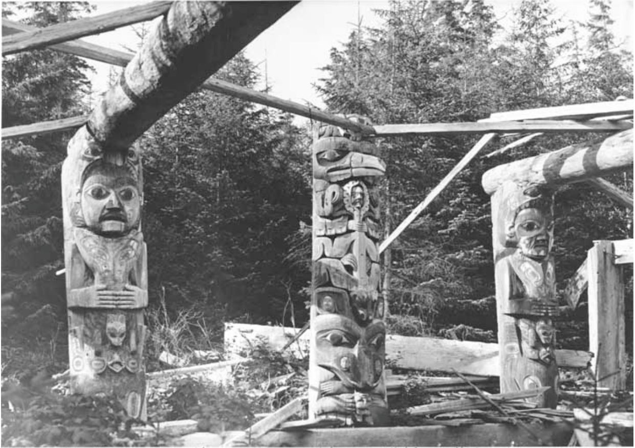
014 Indian Totems which formerly supported roof of Tribal Community House at Kuskoon - K194
